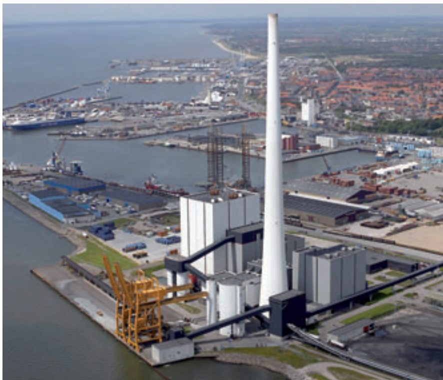
The CO 2 capture industrial pilot unit of the Castor project, coordinated by IFP Energies nouvelles and financed by the European Commission at the Esbjerg power plant (Denmark).
